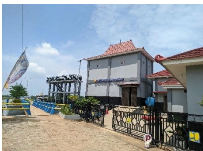
Figure 6. Pump station for preventive measures against the impact of flooding
